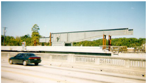
Figure 1 Trunnion-Hub-Girder (THG) assembly.
